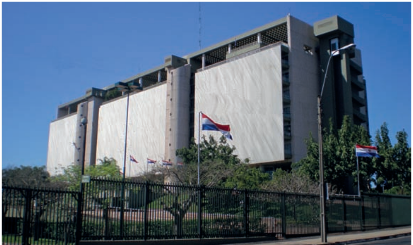
Premises of the Banco Central del Paraguay in the City of Asunción / BCP
