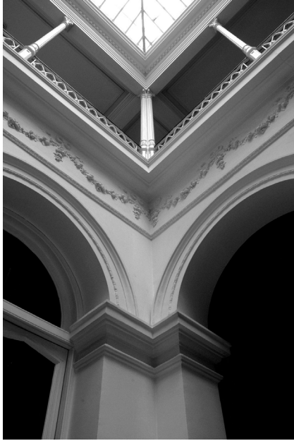
Detail of the interior courtyard in the CEMFI head offices.
