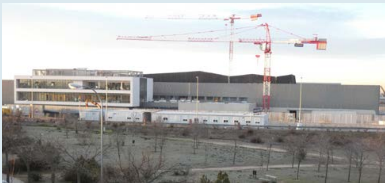
View of the construction site of the new IMBISA printing works.
