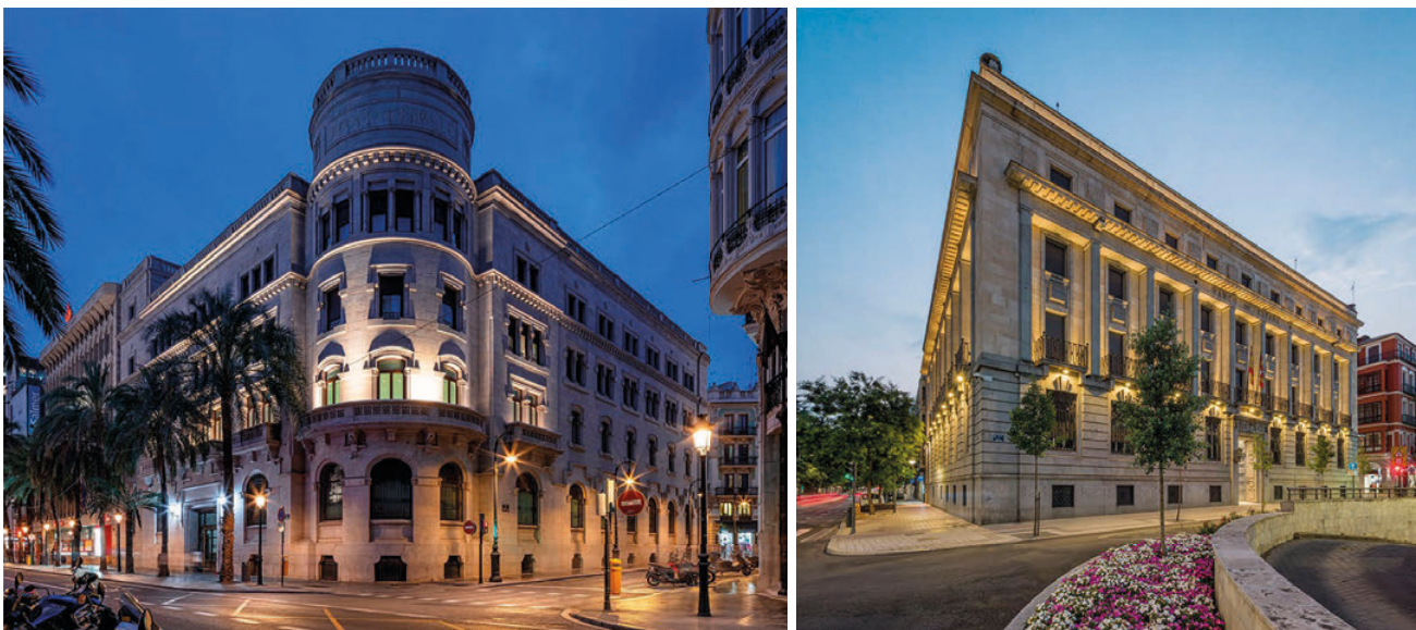
Façades of the València (left) and Valladolid (right) branch buildings.
